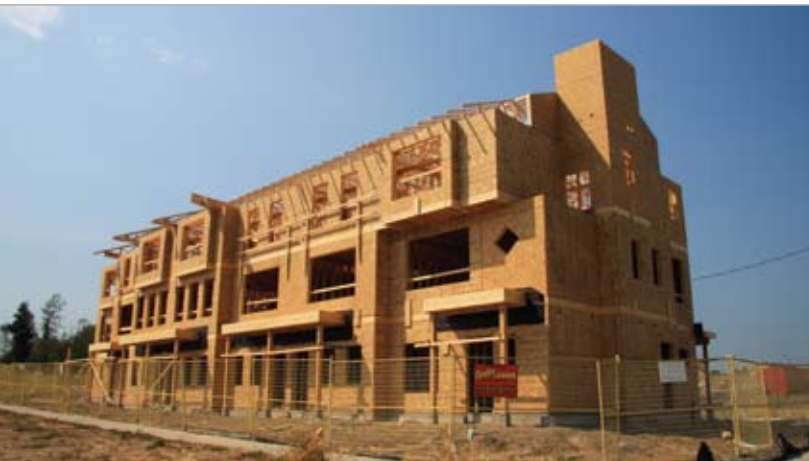
Almost ready for the roof.
