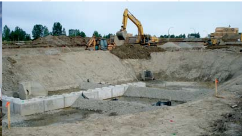
Preparing the retention pond.
