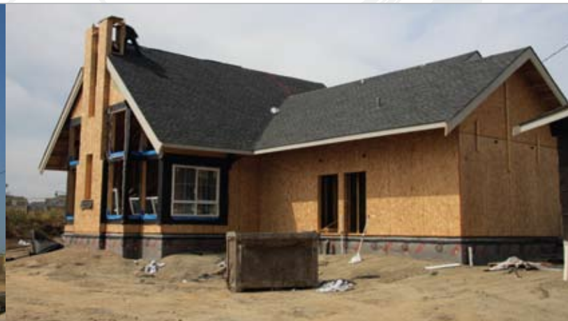
The roof is on The Clubhouse!
